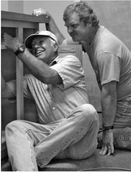
YOTO supporters Andy Fiore and Tim Powell (l to r) volunteered their expertise to install upper and lower cabinetry and a countertop to create needed office storage and workspace.
